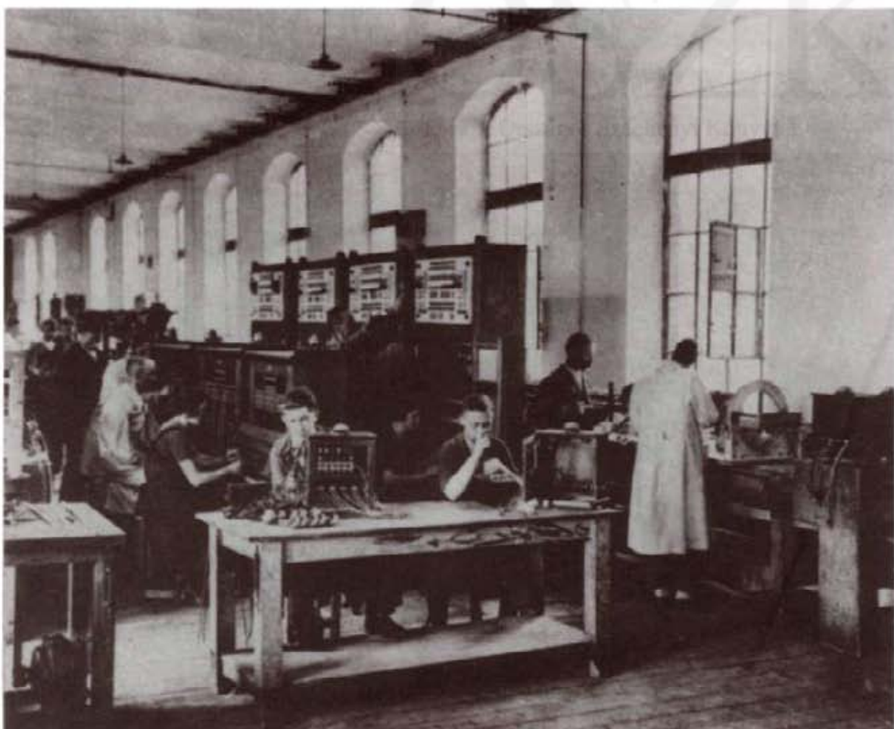
The manual switches of the telephone exchanges were also made here.
