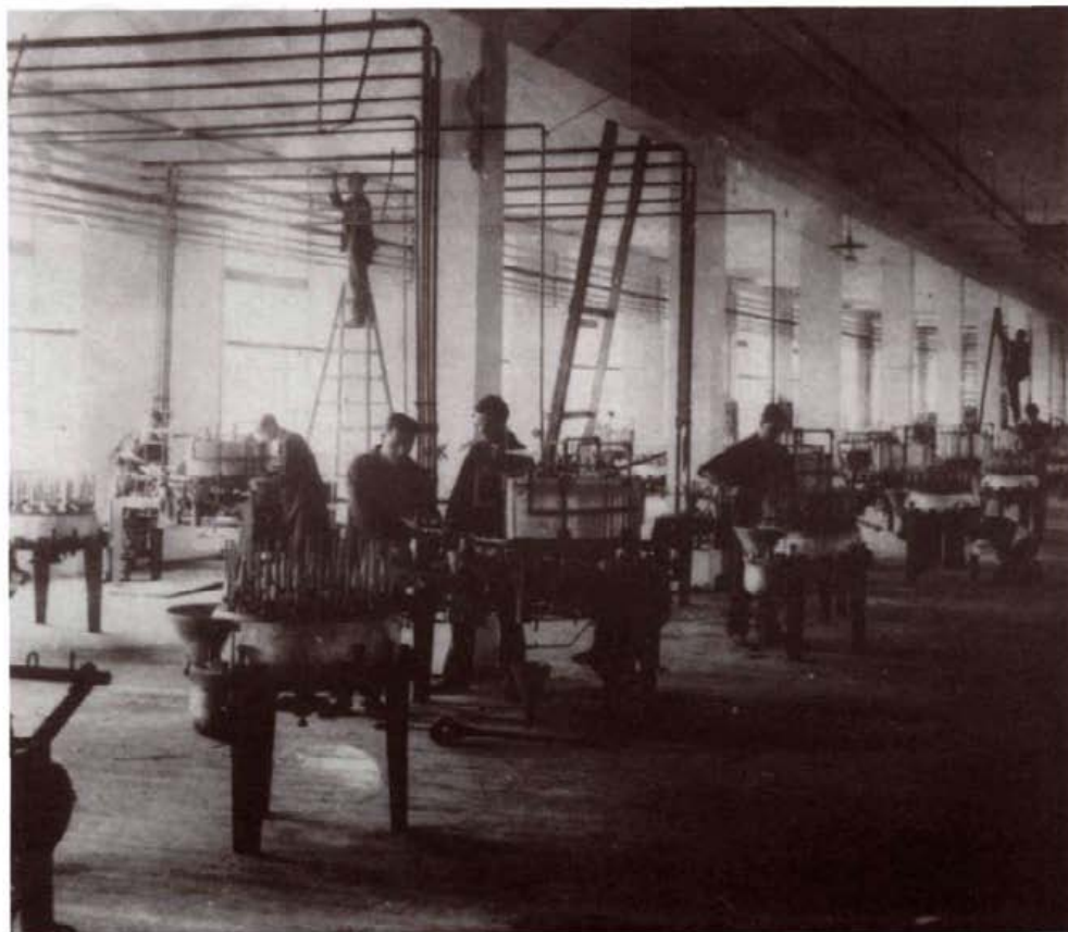
The final touches are being put to the recently finished 'Audion' building at the beginning of the 1930s; the workers are painting the utility system and install the so called "sealex" machines.
